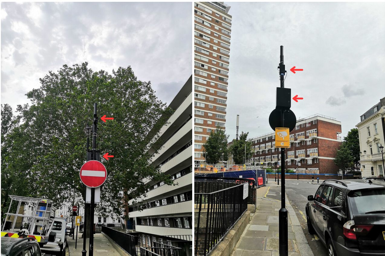
Noise and video monitor attached to the 'no entry' sign post near Q-Park Pimlico's entrance (see arrows).
