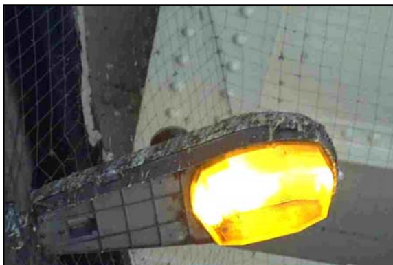
11. Lamp provides pigeon rest, despite netting. Carlisle Lane
