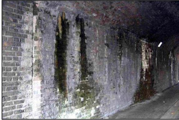
1. Water damage to brick arch and walls Sail Street
