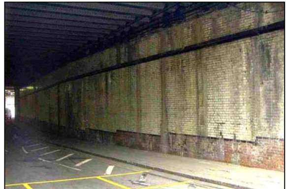
2. Water damage to white tiled sections Addington Street
