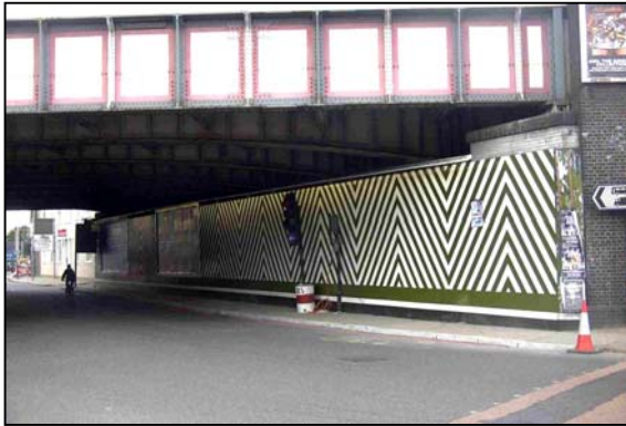
Raised wooden chevron covering walls, reduces graffiti and flyposting Parry Street
