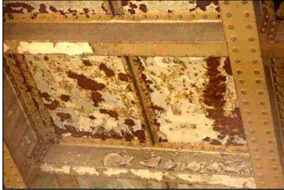
7. Rusting and peeling parapet/ceiling Alaska Street
