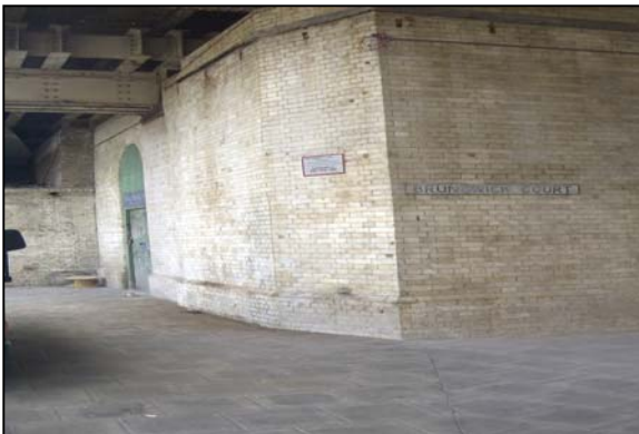
White tiles, cleaned and coated with anti-graffiti treatment Brunswick Court (May 2003)
