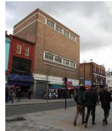
Transport for London building with potential for the installation of a modular green wall
