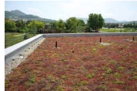
An extensive Sedum roof, comprising a pre-planted mat and shallow substrates (GRC)
