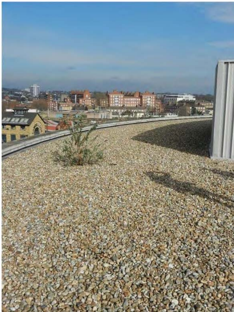
Ice Wharf – Existing
