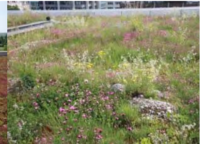
A biodiverse roof with wildflower species adapted to shallow substrates (GRC)
