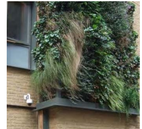
Example of a modular green wall system attached to a wall face.
