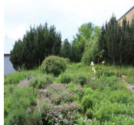
A semi-intensive roof with greater substrate depth and plant diversity (GRC)
