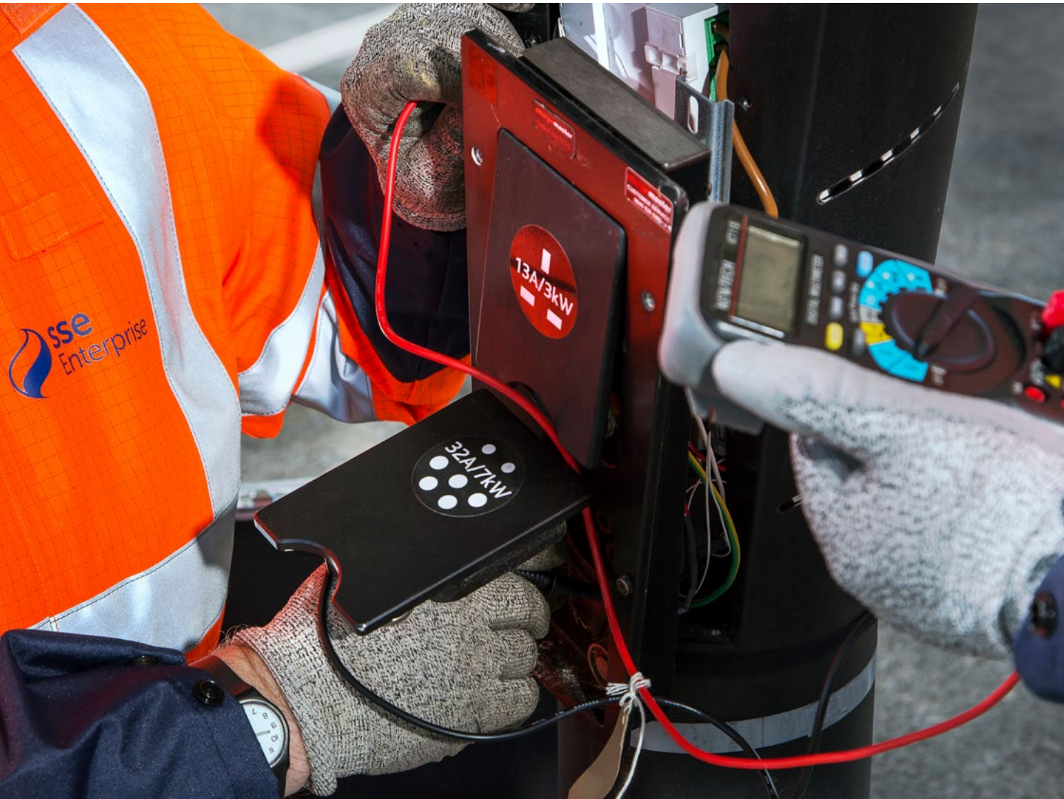
Image 8 Slow charge point being installed in London
