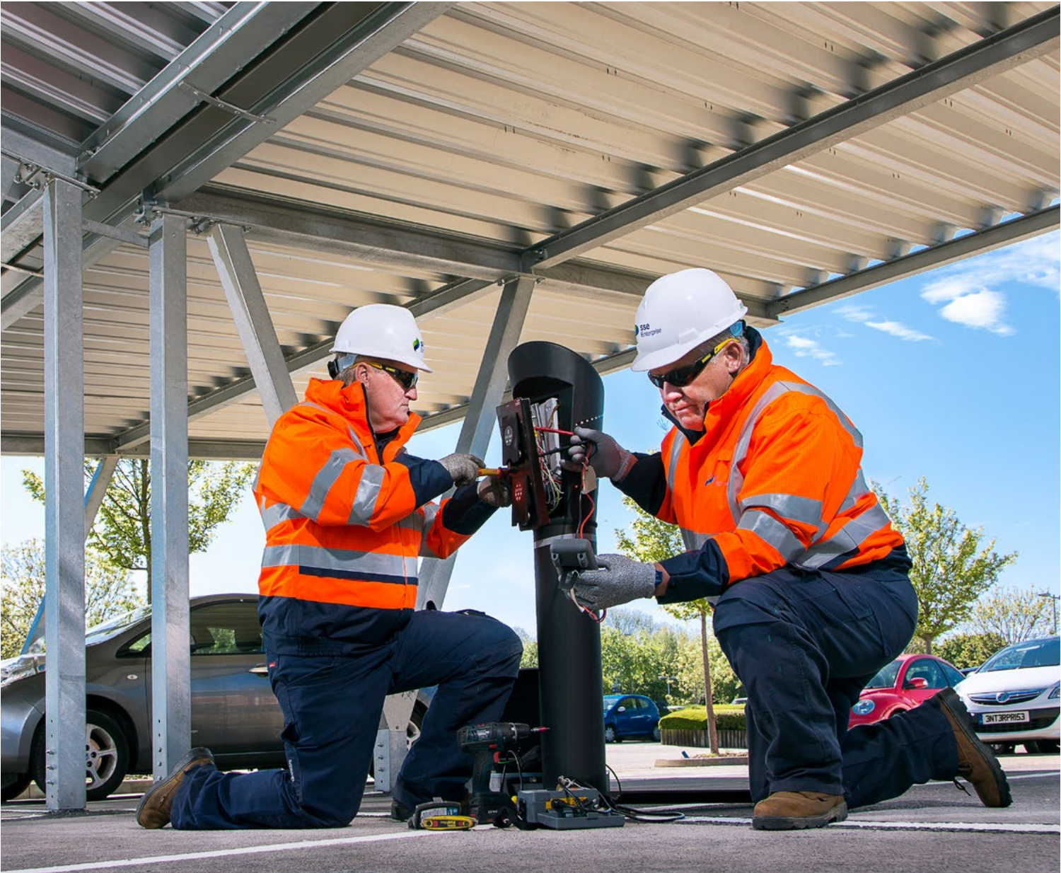
Image 9 Slow charge point being installed in London
