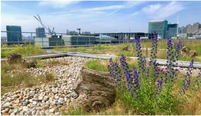
Extensive 'brown' biodiverse green roof, Bishopsgate, London Photo: Dusty Gedge
