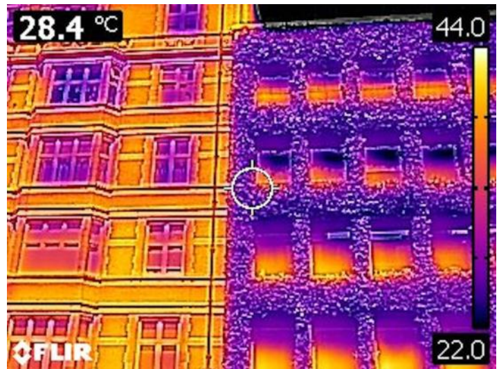
Thermal image showing the surface temperature of a green wall, central London Image: Gary Grant
