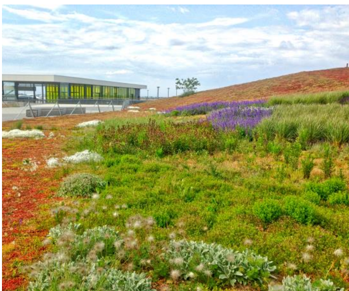
Extensive and semi-intensive green roof on the Emporium Hyllie, Malmö, Sweden Photo: Dusty Gedge
