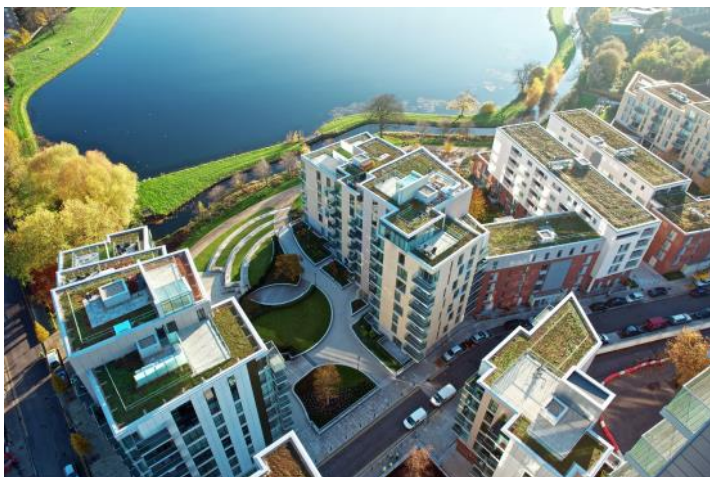
Extensive green roofs, Woodberry Down, north London Photo: Berkeley Homes North East
