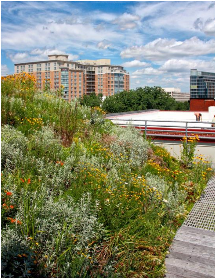
Extensive green roof, Washington, DC, USA.
