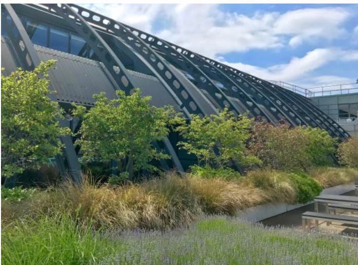
Intensive green roof, Embankment Place, central London Photo: Dusty Gedge
