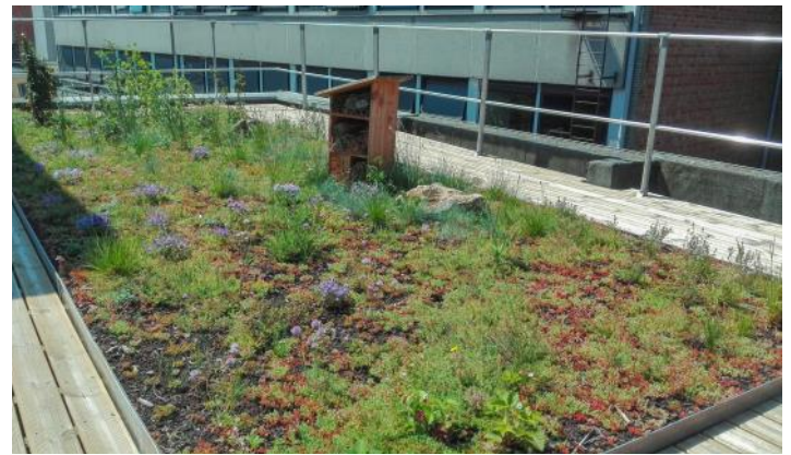
Blue green roof, Antwerp Photo: Vegetal ID
